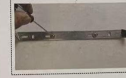
15、The hanging board is locked on the ceiling with screws
